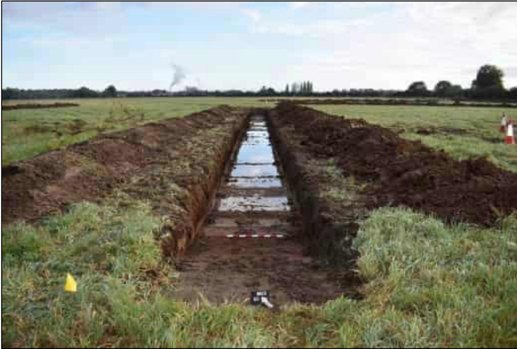
Plate 38: Post-excitation photograph of Trench 0611, looking northeast (Scale: 1m)
